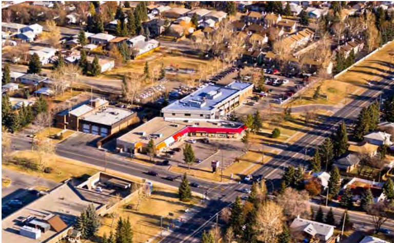
Looking east at the commercial building on the corner of 45 th Street and 17 th Avenue S.W., scheduled for removal in January 2010.
